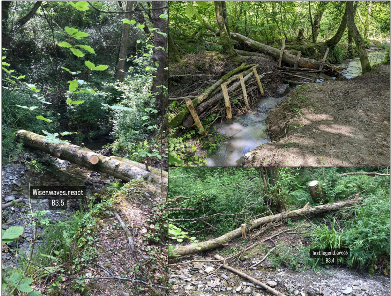
Figure 5. Example of NFM woody dams installed on Bircham Stream © Plymouth Natural Grid. Text refers to what3words locations.
