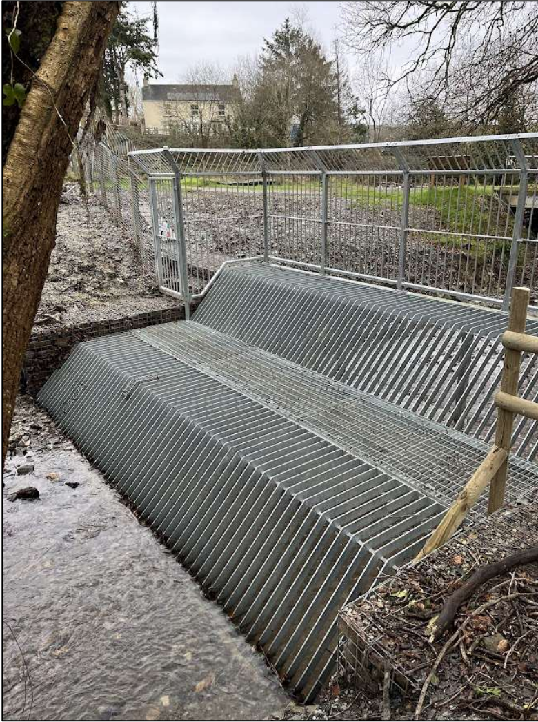
Figure 10. Grill downstream of the beaver enclosure installed in Phase 3, during 2023. Whilst not in itself an NFM intervention it is worth noting the installation of this grill (and a comparative one on the beaver enclosure inflow) could also have an impact upon flow regimes.
